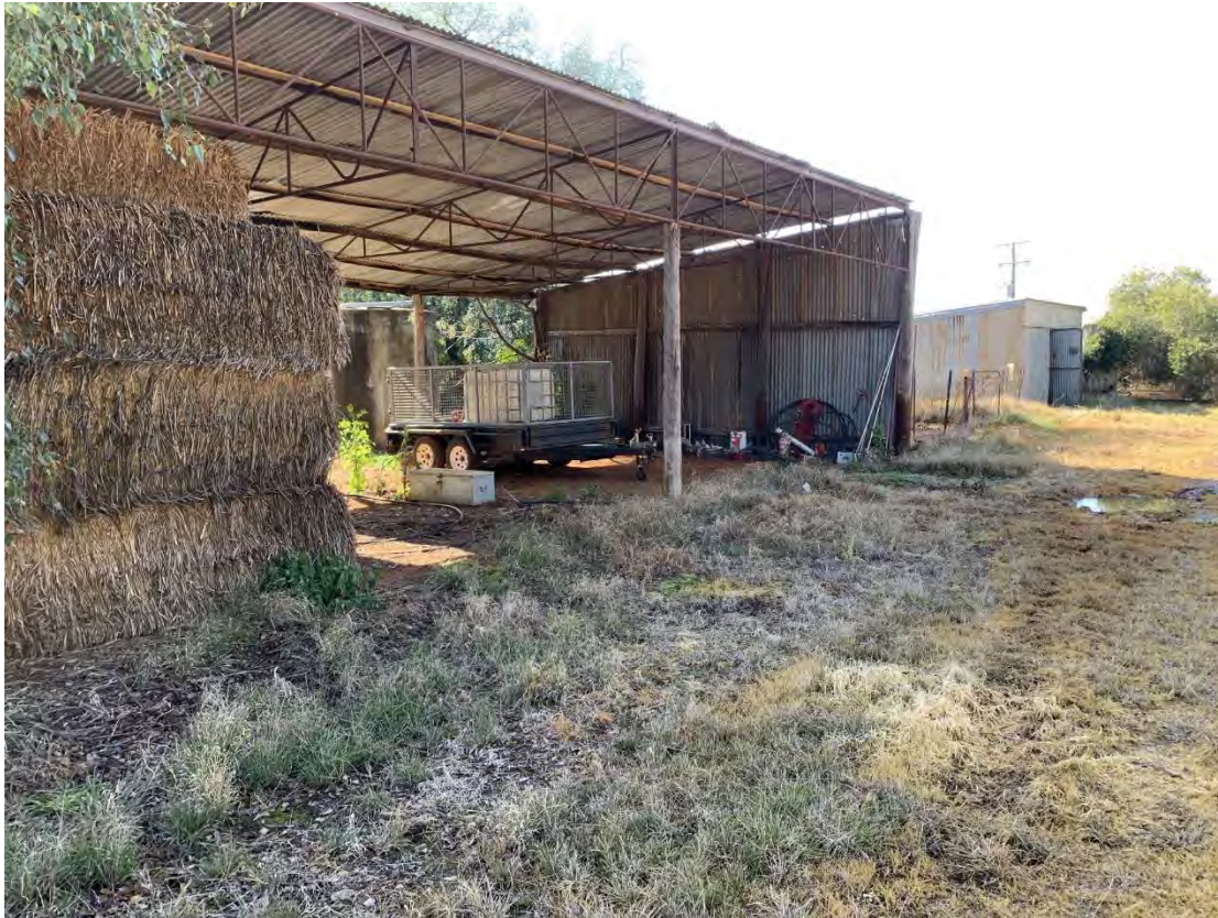
Photograph 13: The wooden framed steel machinery shed.
